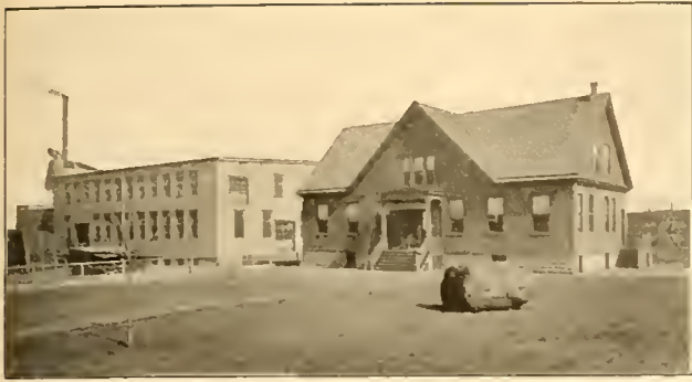
OFFICE AT WEST END, JERSEY CITY.
